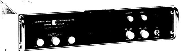
The CEI Type SM-8512 Signal Monitor has been designed for use with receivers having a 455-kc IF center frequency. It provides a visual display of signals in a band around the received frequency.
